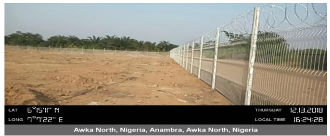
After Site Preparations (Fencing Completed)
