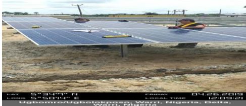
Solar Panels being mounted
