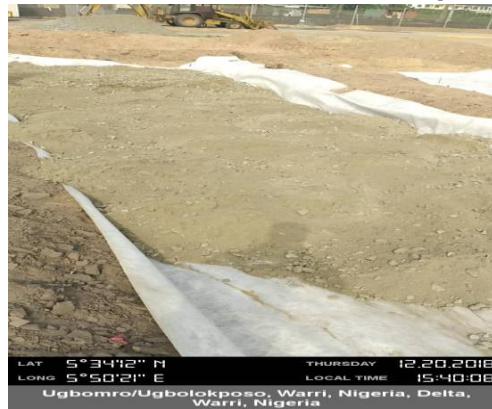
Site Internal Roads Preparations
