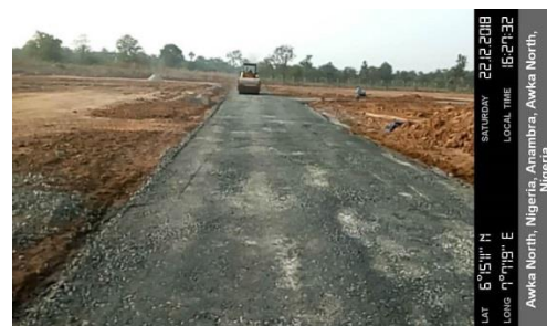
Internal Roads Preparations
