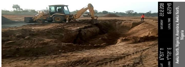
Equipment Foundation Works
