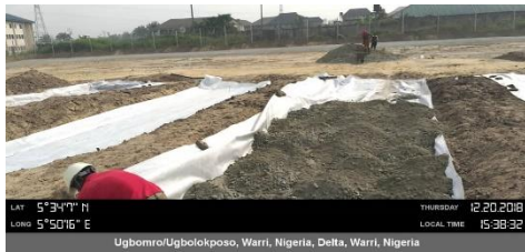
Equipment Foundation Works
