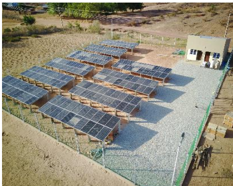
Aerial Vie of Commpleted 60kW Power Plant
