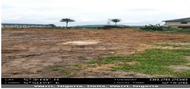
Before Site Preparations
